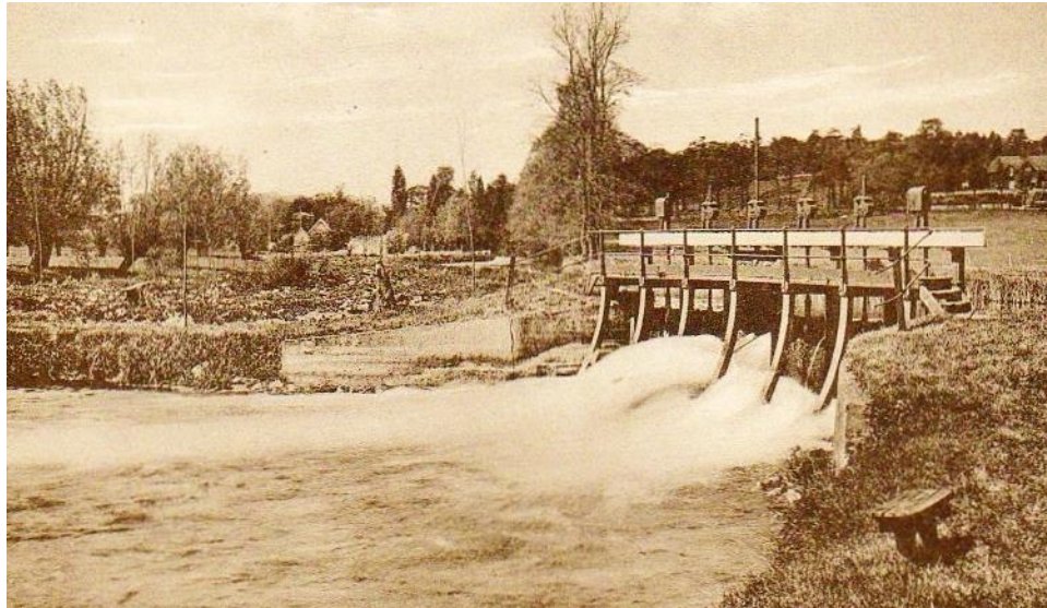
The six gates weir which for most of the C20th allowed surplus water to flow from the Millstream in to the Old River Lea via a spillway. This was located at or close to the location of the 1743 spillway shown on the Whittenbury's Turnpike map above.
