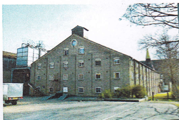
Brown Malting with unusual shaped kiln at rear. Grain intake can be seen centre left.
