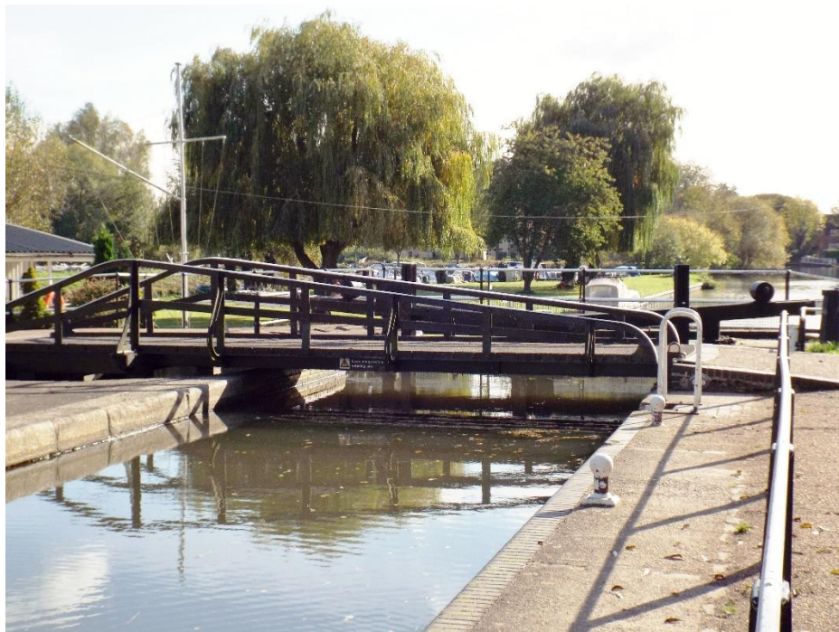
An unusual feature of Stanstead Lock is the swing bridge which today provides access to the cruising club located on the north side of the navigation
