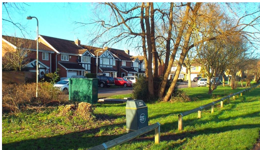
The above image taken from the river tow path showing some of the homes in Lawrence Avenue that enjoy the benefit of facing onto the River Lea Navigation.
